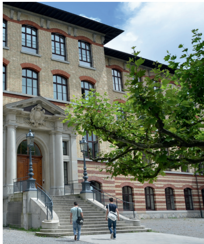
The department's main building, CAB, was originally built in 1886 to house ETH's chemistry department. The listed building retains much of its original character, including the historic chemistry lab, which has been preserved and serves as a study space today.
